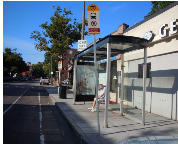
Custom designed shelter design with the side glass panel omitted in Boston, MA due to the proximity of the shelter to the curb
