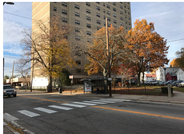
Mid-block RIPTA stop at Providence Housing Authority’s Carroll Towers, at Smith Street at Common Street in Providence, RI
