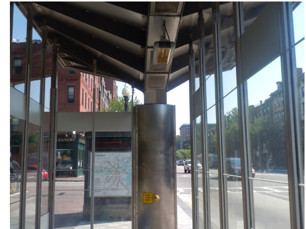
Heated shelter along MBTA's Silver Line in Boston, MA
