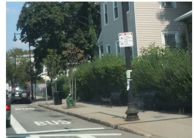
Overgrown shrubs overhang benches at an MBTA bus stop
