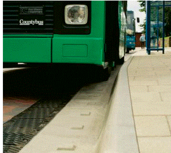
Marshalls "Bus Stop Kerb" with channel unit
