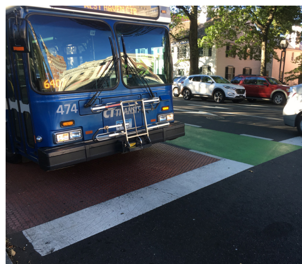
Bus stop in New Haven, CT has a stamped colored asphalt treatment
