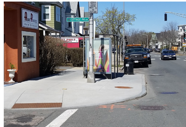
Near-side curb extension with realigned curb ramp at an MBTA bus stop in Cambridge, MA
