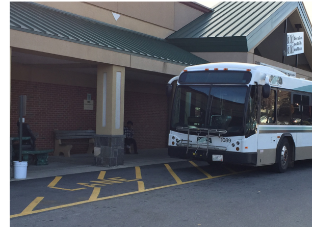
RIPTA stop at East Side Market in Providence, RI lacks any curb reveal at the sidewalk edge
