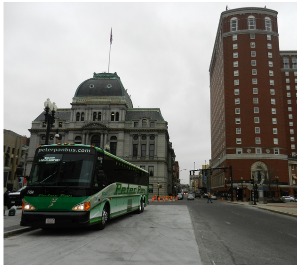
Concrete bus pad at the former Peter Pan stop on Washington Street at Kennedy Plaza in Providence, RI
