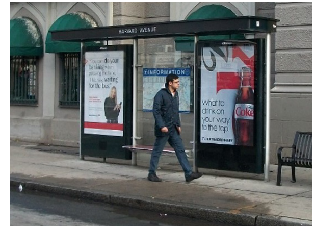
Narrow shelter design with no side panels in Boston, MA
