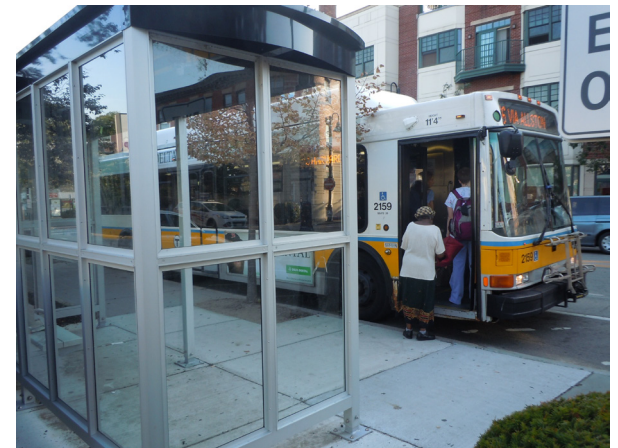
Standard shelter size with a rear and two side panels in Brookline, MA
