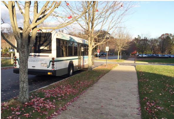
RIPTA stop at Bryant University in North Smithfield, RI has a grass strip in the landing area
