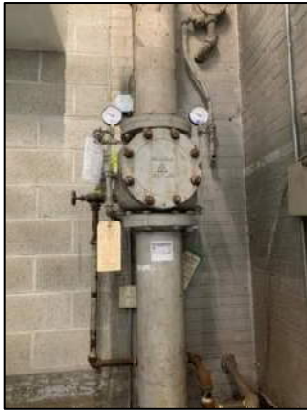
Figure 44: Fire Sprinkler Riser in Boiler Room
