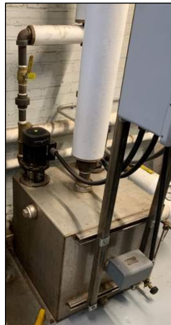
Figure 27: Condensate Receiver in the Boiler Room
