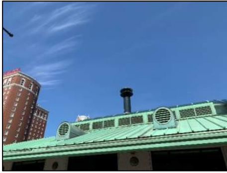
Figure 7: Boiler Exhaust and Louvered Exterior for Mechanical Space
