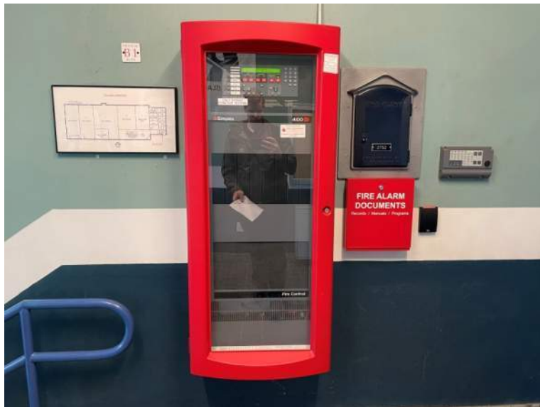
Figure 1: Fire Alarm System
