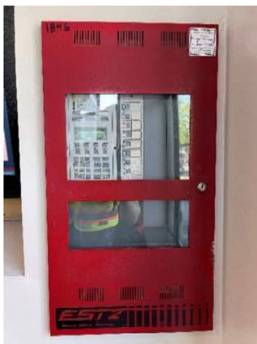
Figure 1: Fire Alarm Control Panel
