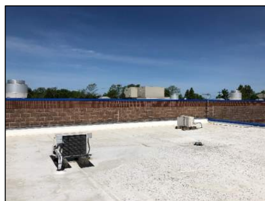
Figure 9: Split System Condensers
