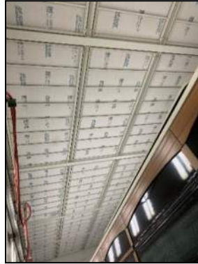
Figure 34: Paint Booth Exhaust (Interior to Booth)
