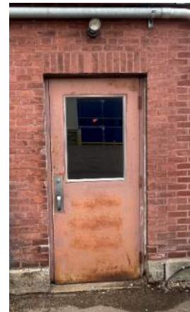
Figure 8: Emergency remote head
