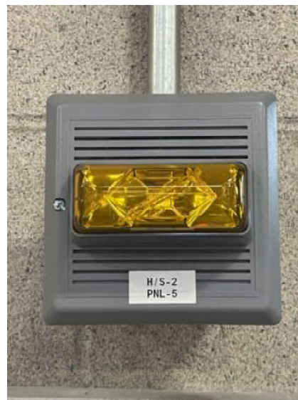
Figure 2: Amber Strobe for CO detection system
