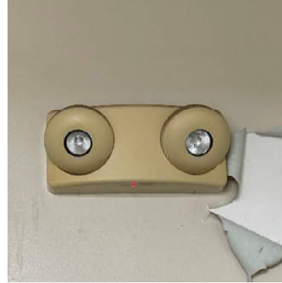
Figure 6: Emergency Battery Unit
