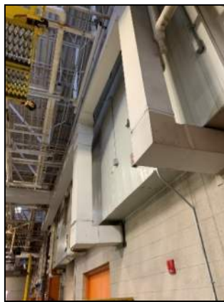
Figure 24: MAU Ducting from Garage to Surrounding Rooms
