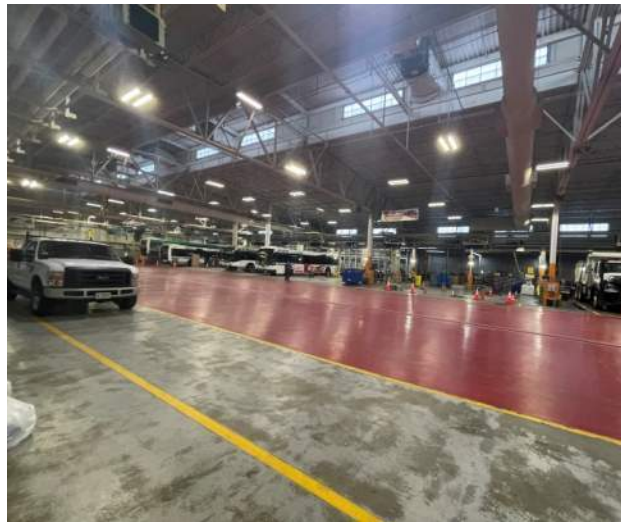
Figure 2: LED High-bay and fluorescent fixtures
