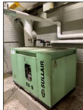
Figure 18: Air Compressor
