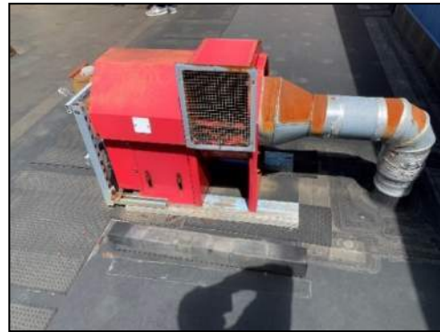
Figure 29: Exhaust Fan on the Roof
