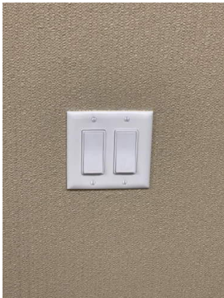
Figure 7: Toggle switches
