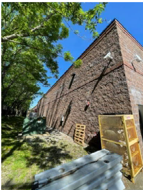
Figure 9: Exterior Wall packs
