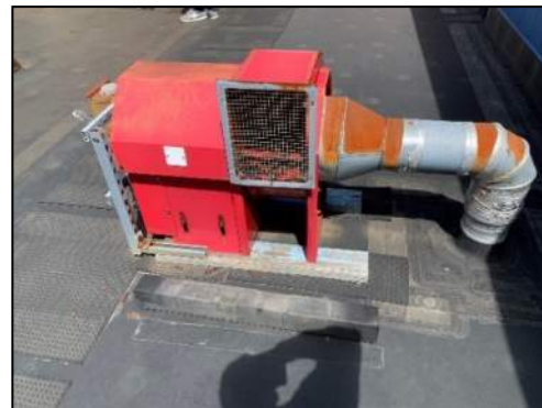
Figure 29: Exhaust Fan on the Roof
