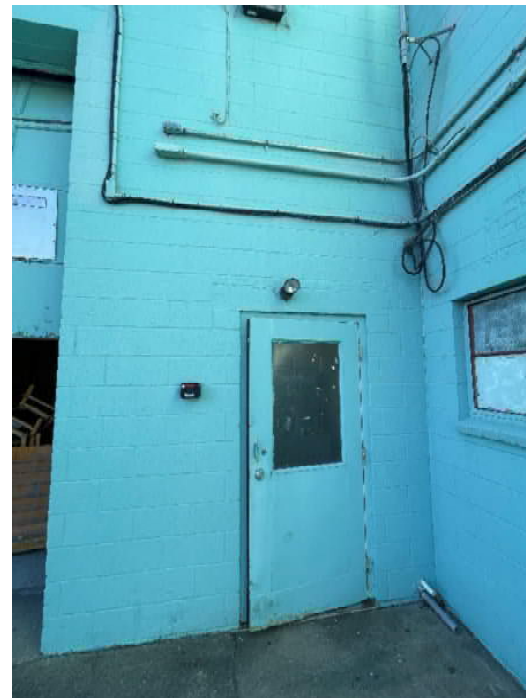
Figure 10: Emergency remote heads
