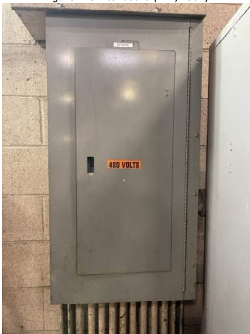
Figure 3: Abandoned/Damaged Panelboard
