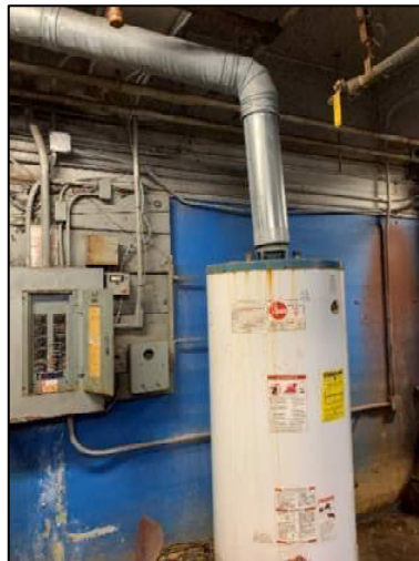
Figure 5: Abandoned Gas-Fired Water Heater in Abandoned Boiler Room
