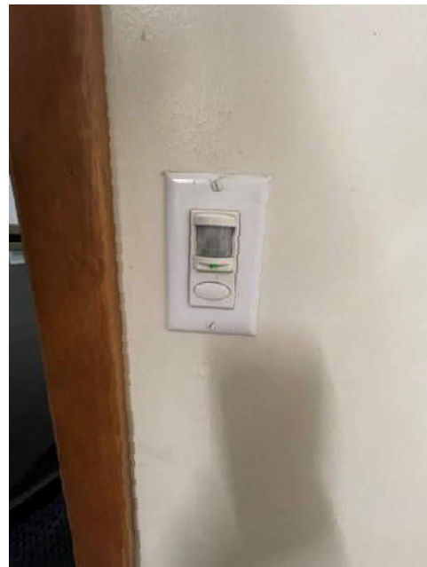
Figure 8: Wall switch occupancy sensor
