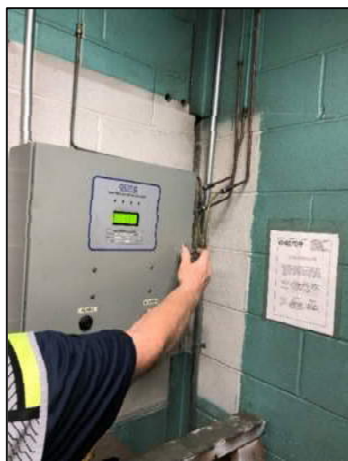
Figure 20: NO2 and CO2 Control Panel
