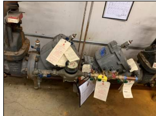
Figure 43: Double-Check Valve Assembly
