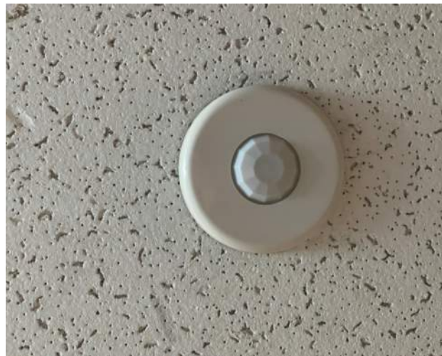
Figure 4: Ceiling mounted occupancy sensor
