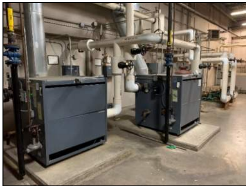
Figure 18: Hydronic Heating System Boilers
