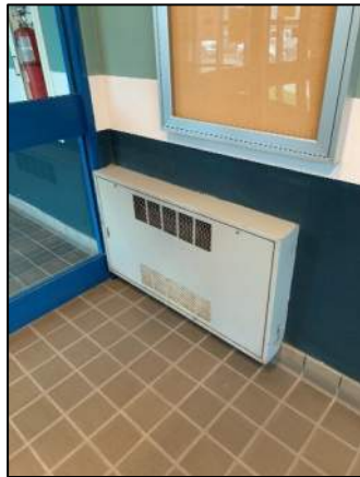
Figure 26: Panel Radiator
