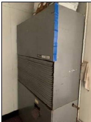
Figure 37: Indoor Evaporator
