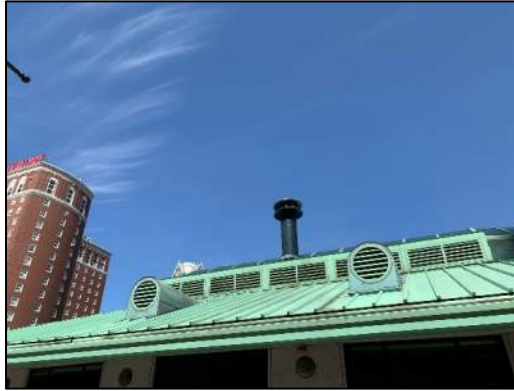
Figure 22: Boiler Exhaust and Louvered Exterior for Mechanical Space
