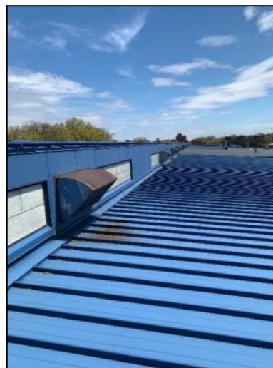
Figure 31: Exhaust Fan Terminals on Peak of Roof
