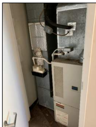
Figure 15: Indoor Evaporator with Gas-Fire Furnace
