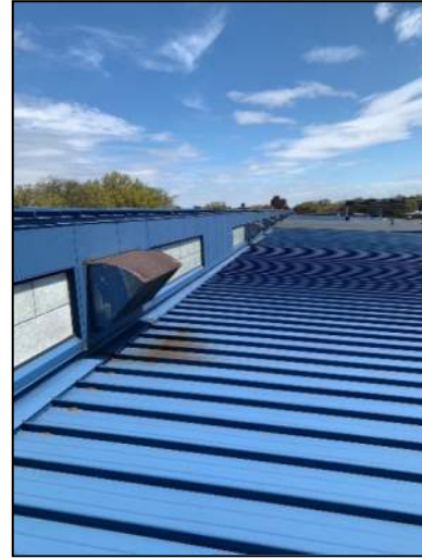
Figure 31: Exhaust Fan Terminals on Peak of Roof
