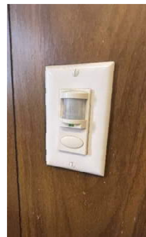
Figure 4: Wall switch occupancy sensor
