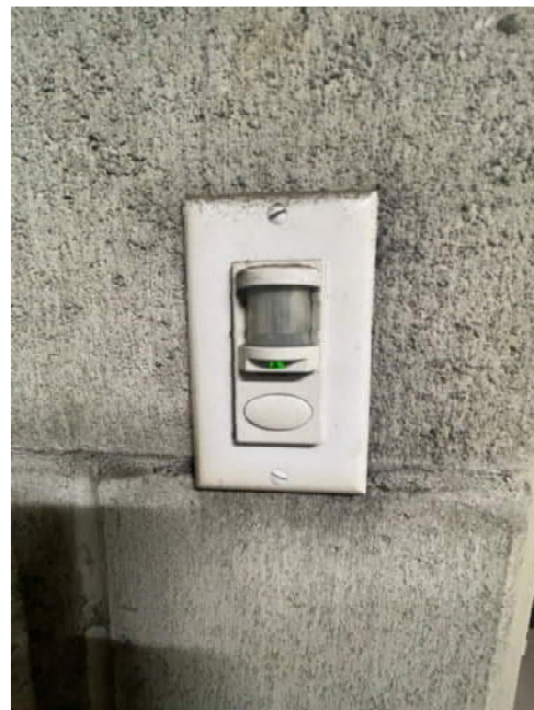
Figure 8: Wall switch occupancy sensor
