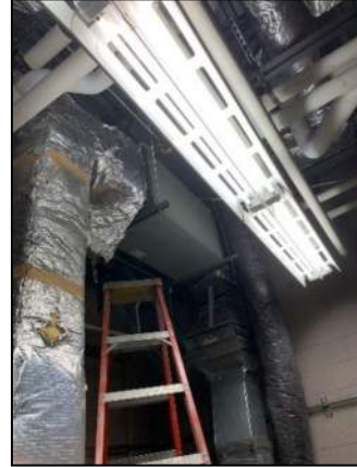
Figure 38: AC Fan Coil Unit
