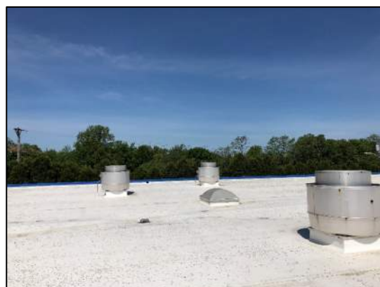
Figure 17: Centrifugal Upblast Exhaust Fans
