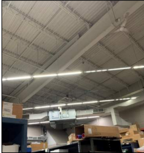
Figure 20: Fan Coil Unit in Parts Storage
