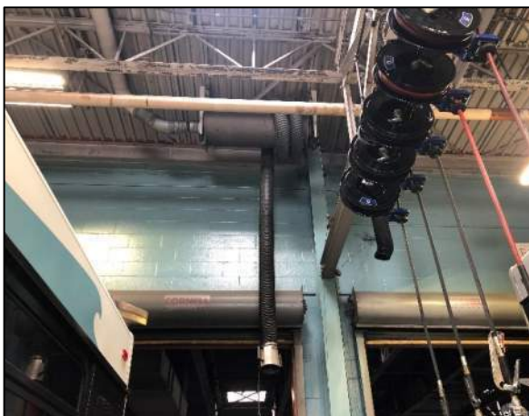
Figure 14: Rope-and-Pulley Exhaust System
