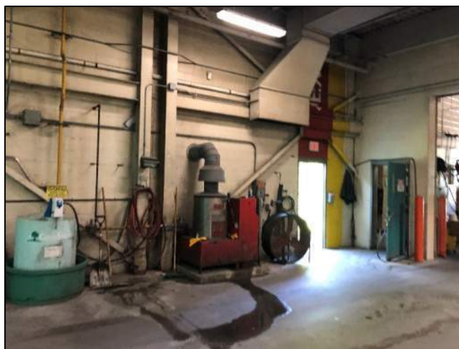
Figure 5: Dedicated Boiler for Bus Wash
