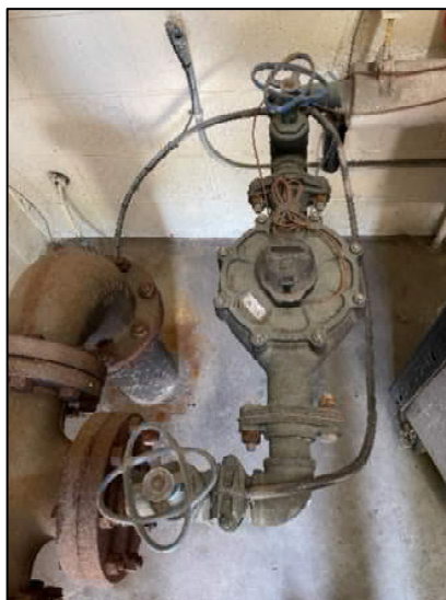
Figure 3: Domestic Water Meter
