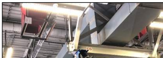
Figure 15: Ceiling Mounted Exhaust Fan
