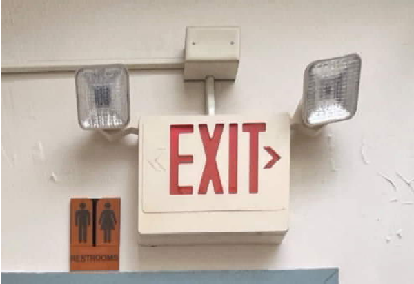
Figure 5: Unilluminated Exit sign
