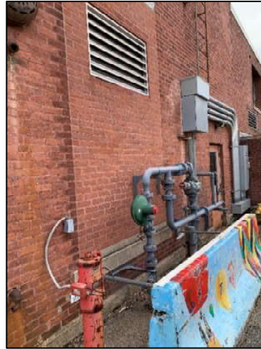
Figure 43: Post Indicator Valve
