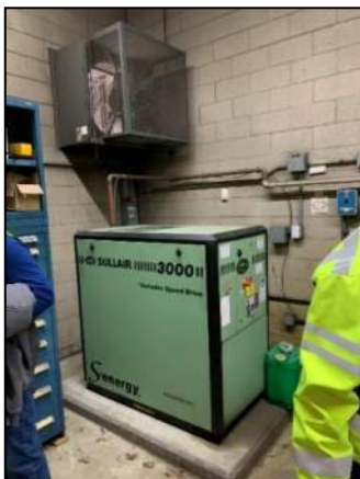
Figure 14: Air Compressor
