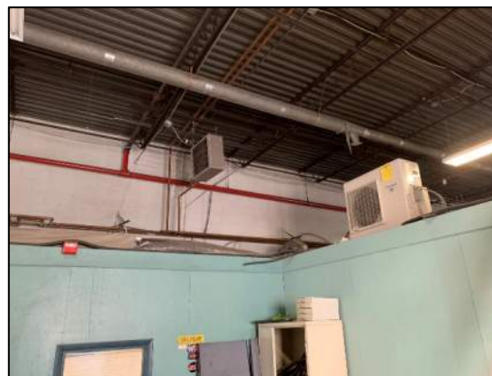
Figure 18: Mini-Split Condenser on Roof of Shop Office
