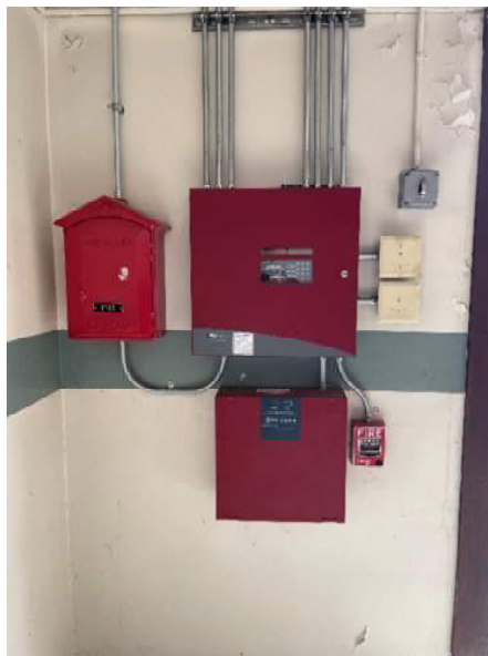
Figure 52: Fire Alarm System
