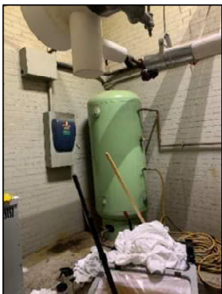
Figure 16: Compressed Air Tank
