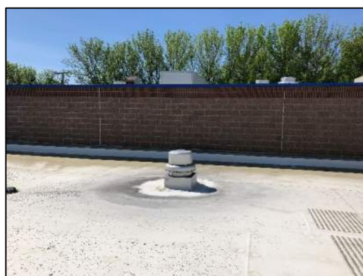
Figure 18: Centrifugal Downblast Exhaust Fans
