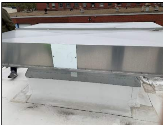
Figure 39: Makeup Air Unit Termination
