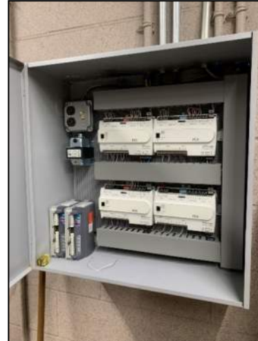
Figure 45: Working BMS Control Panel in Boiler Room
