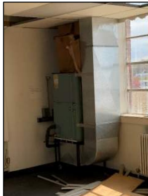
Figure 38: Indoor Evaporator
