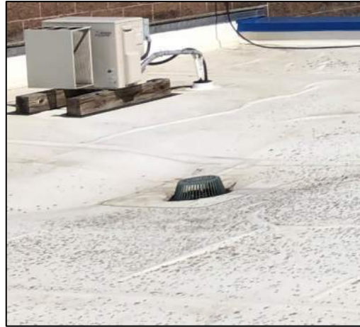
Figure 7: Roof Drain
