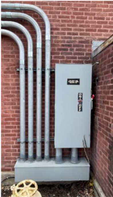
Figure 1: Main Service Disconnect
