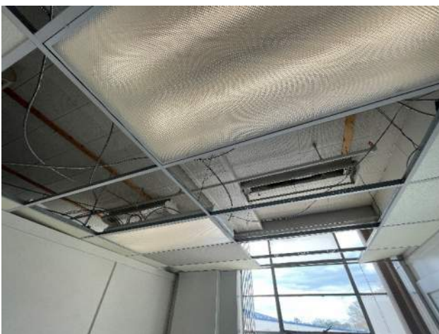
Figure 3: Existing and abandoned fluorescent fixtures
