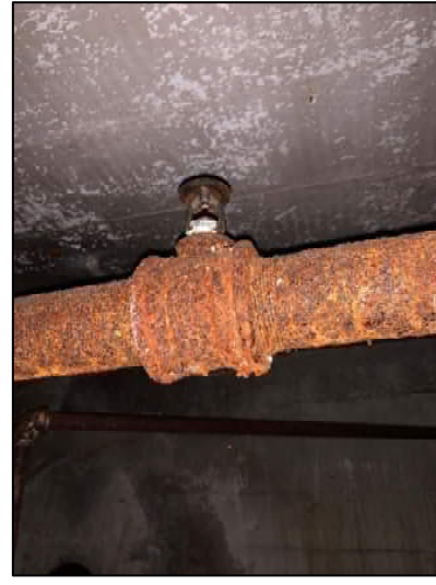
Figure 49: Rusty Fire Sprinkler Line, Basement
