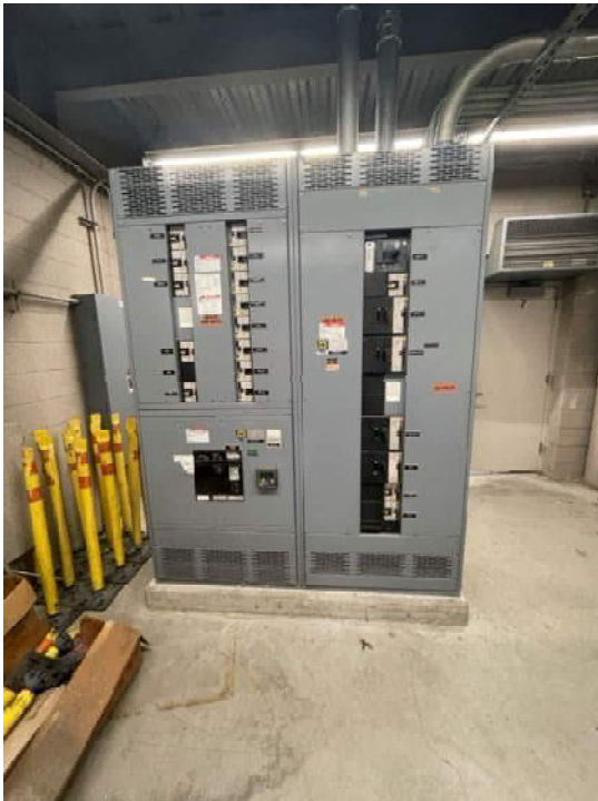
Figure 1: Switchboard (277/480V)
