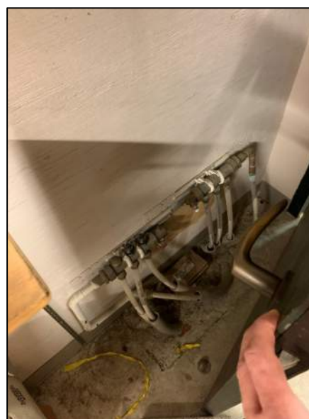
Figure 21: Abandoned Snow Melt Manifold
