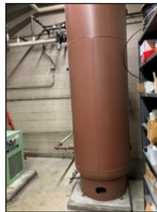
Figure 16: Compressed Air Tank
