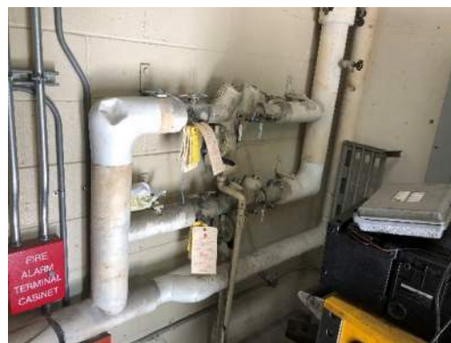
Figure 2: Domestic Water Service Backflow Devices
