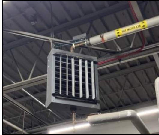
Figure 25: Hot-Water Unit Heater
