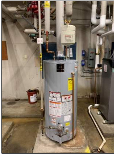
Figure 4: Gas-Fired Water Heater for Office Area
