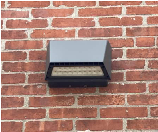
Figure 7: Exterior Wall packs
