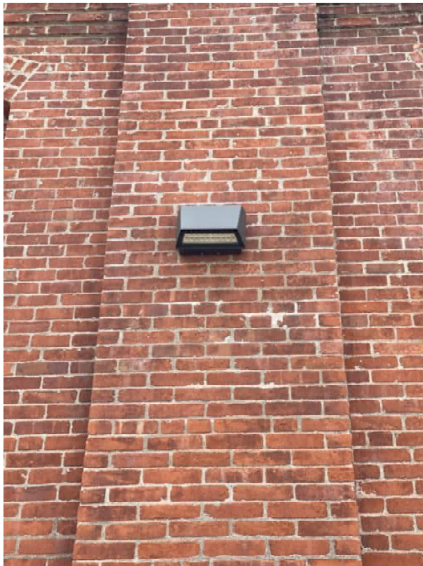
Figure 9: Exterior Wall pack
