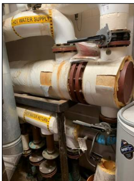
Figure 20: Capped Lines for Heat Exchanger for Abandoned Snow Melt System
