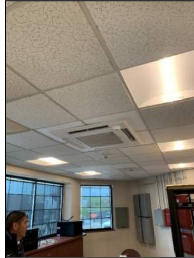
Figure 41: VRF Evaporator for Security Room
