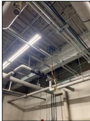
Figure 3: Press-Connect Fittings on a Recently Installed Roof Hydrant
