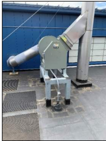
Figure 28: Exhaust Fan on the Roof
