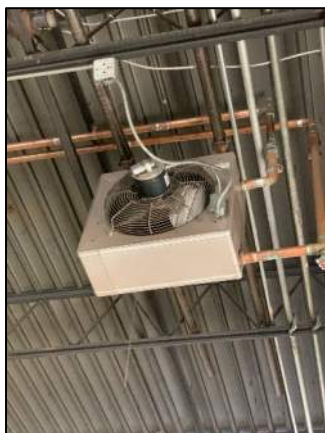
Figure 13: Hydronic Unit Heater
