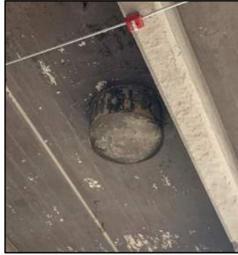
Figure 31: Garage Exhaust Duct Closed
