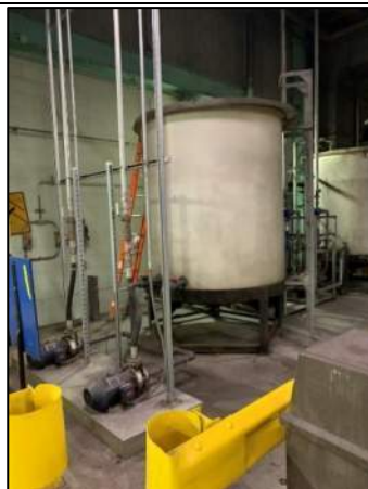
Figure 16: Bus Wash Reclamation System
