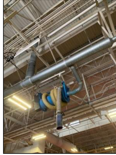
Figure 27: Localized Exhaust System Hose Reel
