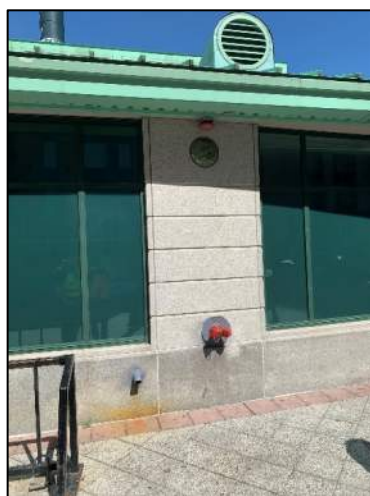
Figure 23: Fire Department Connection and Bell
