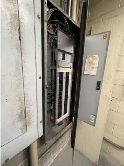
Figure 3: Deteriorating/Damaged Panelboard
