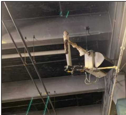
Figure 22: Steam Fan Coil in Garage
