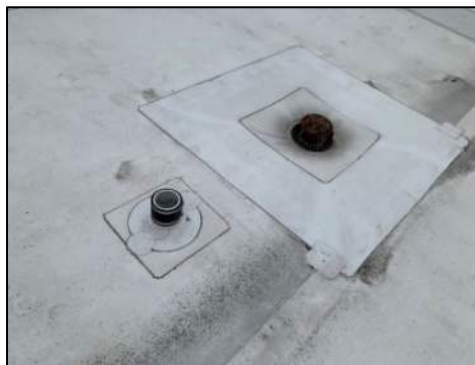
Figure 11: Added Secondary Drain Next to a Primary Drain
