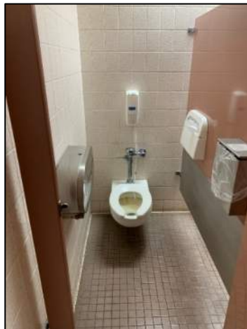
Figure 8: Manual Operated Water Closet
