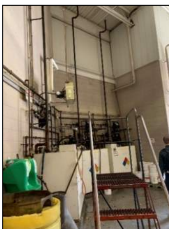
Figure 17: Air-Operated Diaphragm Pumps in Lube Room
