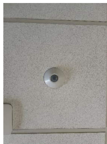
Figure 4: Ceiling mounted occupancy sensor
