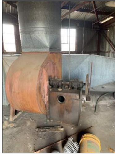
Figure 28: Abandoned Air Handler for Spray Booth, Located on Roof
