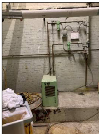
Figure 17: Compressed Air Filter
