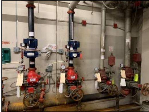
Figure 44: Risers Off of Fire Service Mains
