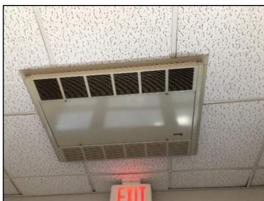
Figure 11: Electric Unit Heater at Entrance
