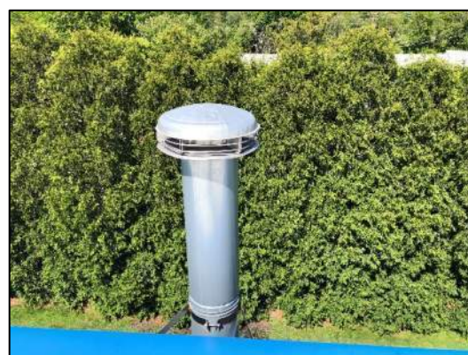
Figure 19: Boiler Exhaust Stack
