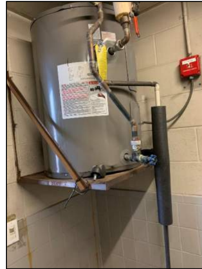
Figure 5: Electric Water Heater for Garage Fixtures
