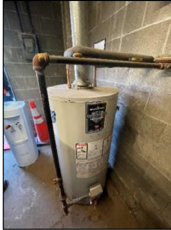
Figure 3: Gas-Fired Tank Water Heater
