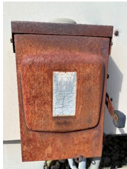
Figure 4: Abandoned equipment/disconnect
