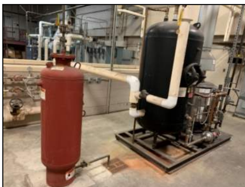
Figure 2: Domestic Water Boiler and Storage Tank
