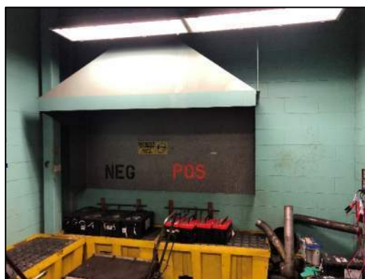
Figure 22: Battery Exhaust Hood
