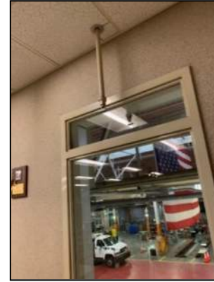
Figure 52: Window Sprinklers in Breakroom
