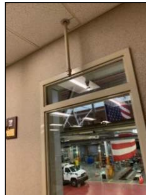
Figure 52: Window Sprinklers in Breakroom
