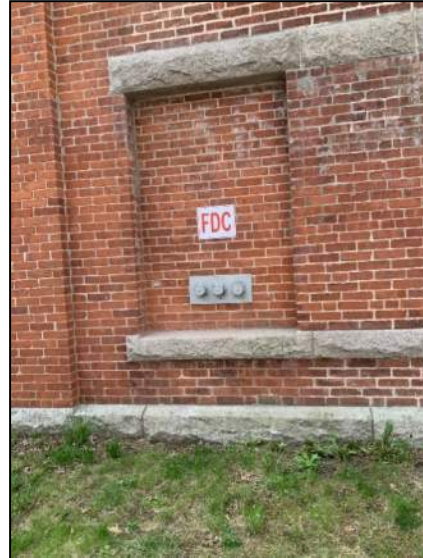
Figure 47: Fire Department Connection
