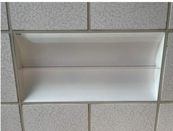
Figure 3: LED 2'X2' troffer fixtures
