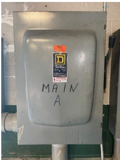
Figure 3: Main Disconnect
