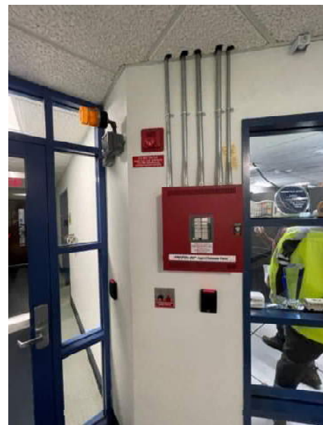
Figure 2: Fire Suppression System
