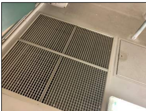
Figure 15: Ducted Floor for Liebert Unit in IT Room
