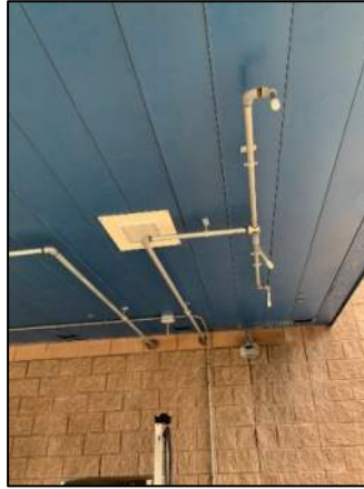
Figure 48: Dry-Chemical Suppression System
