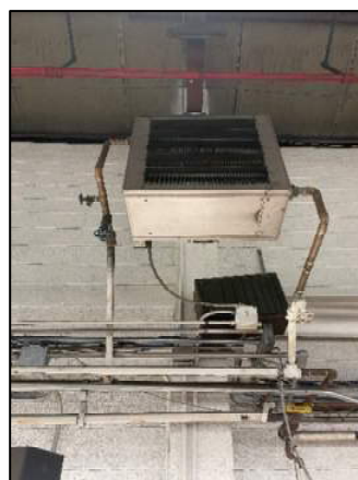
Figure 14: Hydronic Unit Heater
