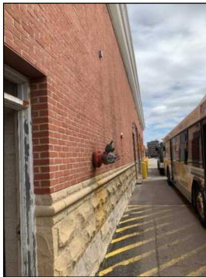
Figure 48: Hose Station Exterior to the Water Room
