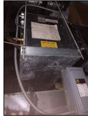
Figure 8: Unitary Air-Conditioning Unit in Attic Above Boiler Room
