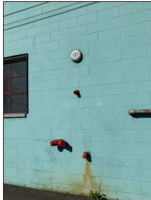
Figure 24: Alarm Bell and Fire-Department Connection
