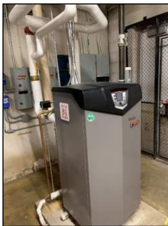
Figure 22: Hydronic Heating System Boiler
