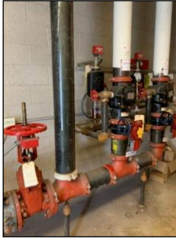
Figure 49: Fire Sprinkler Risers
