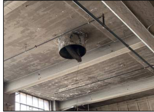
Figure 32: Garage Exhaust Duct Open
