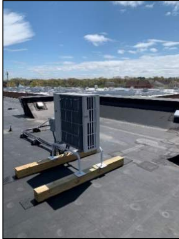
Figure 40: VRF Condenser for Security Room
