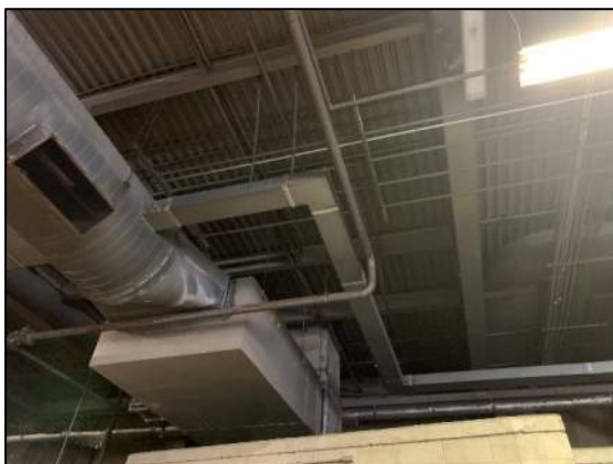
Figure 40: MAU Ducting to Other Spaces
