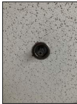
Figure 50: Recessed Sprinkler in Office
