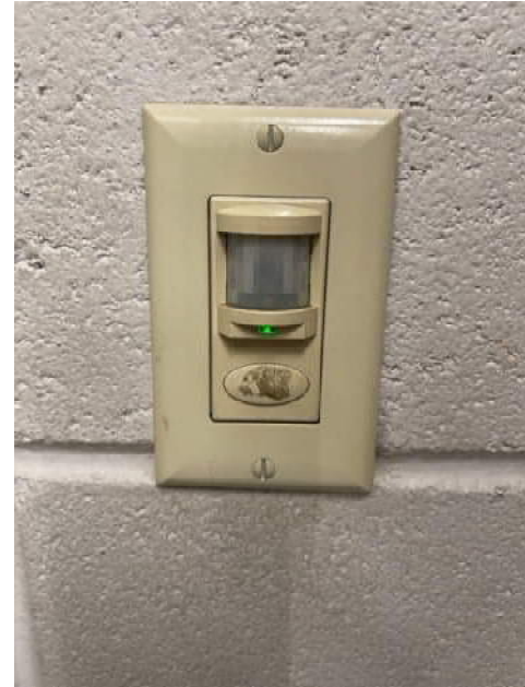
Figure 8: Wall switch occupancy sensor
