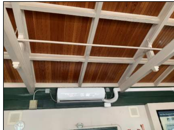
Figure 10: Indoor Unit for Large Waiting Room
