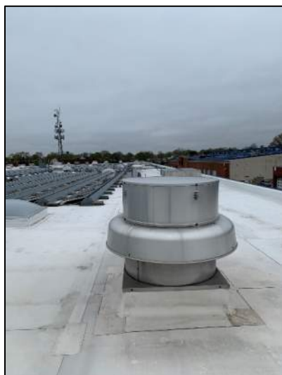
Figure 36: Centrifugal Down-blast Exhaust Fan
