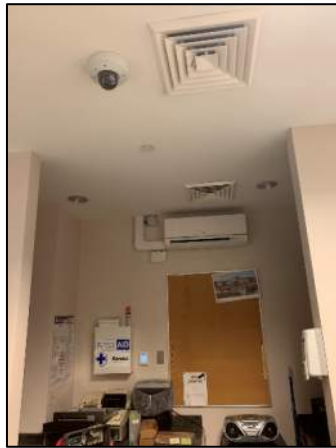
Figure 11: Indoor Unit for Ticket Office
