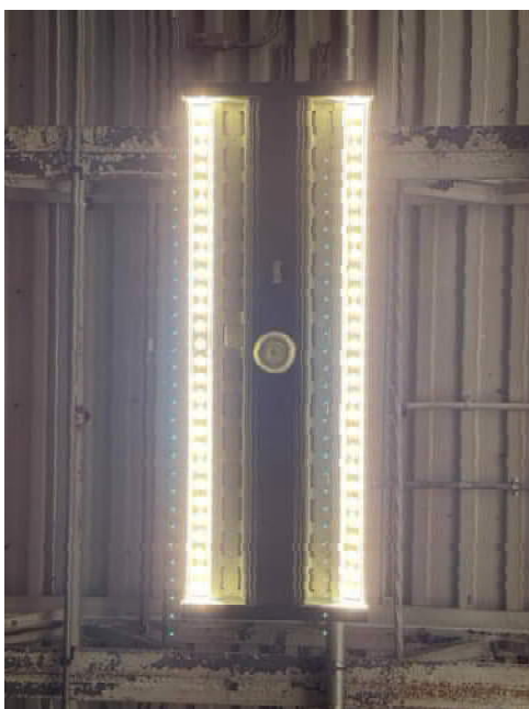
Figure 1: LED High-bay fixtures with integral occupancy sensor
