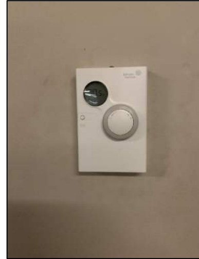
Figure 29: Thermostat for a Zone in the Office
