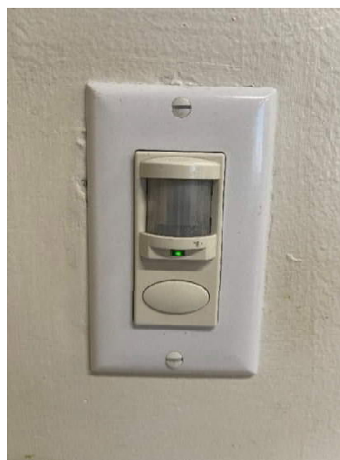
Figure 8: Wall switch occupancy sensor
