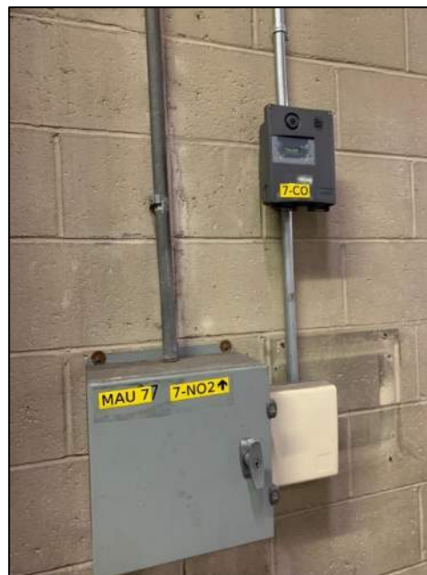
Figure 41: CO and NO 2 Controls
