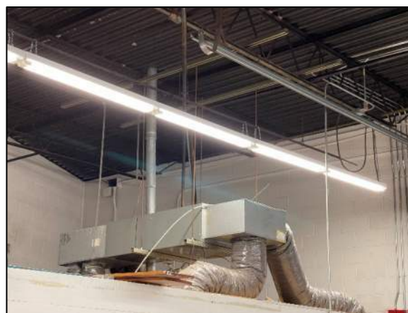
Figure 16: Abandoned Indoor Evaporator
