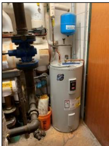
Figure 2: Electric Water Heater
