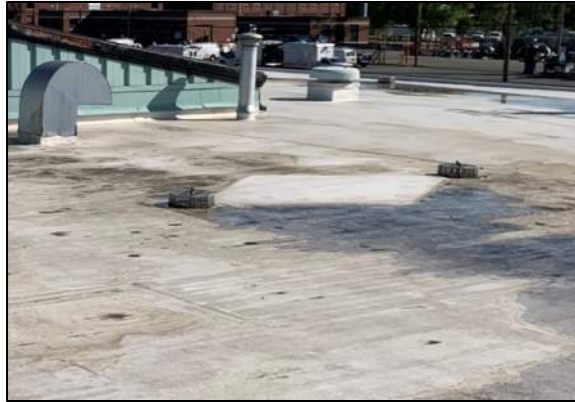
Figure 6: Roof Drains
