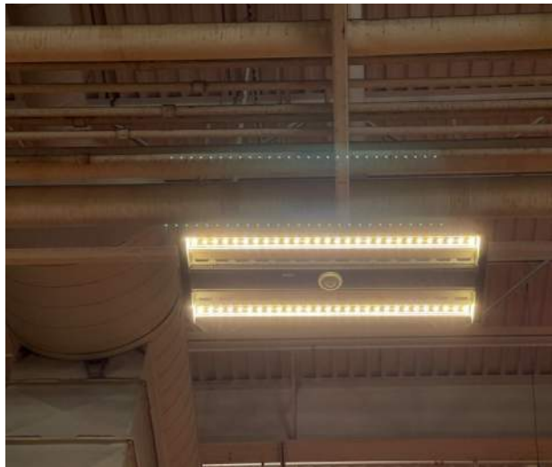
Figure 1: LED High-bay fixtures with integral occupancy sensor
