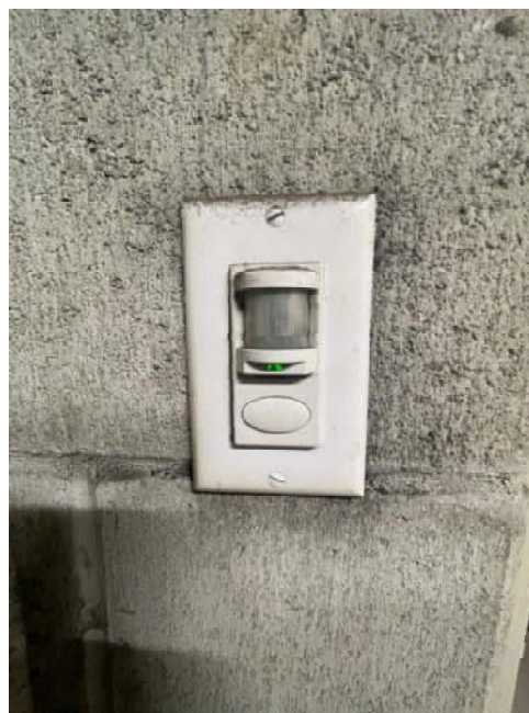
Figure 8: Wall switch occupancy sensor
