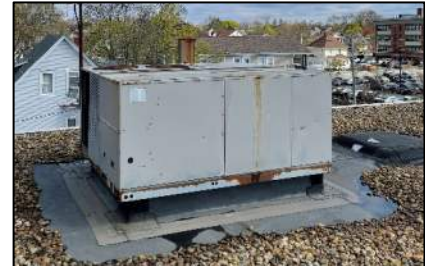
Figure 36: Abandoned Rooftop Unit
