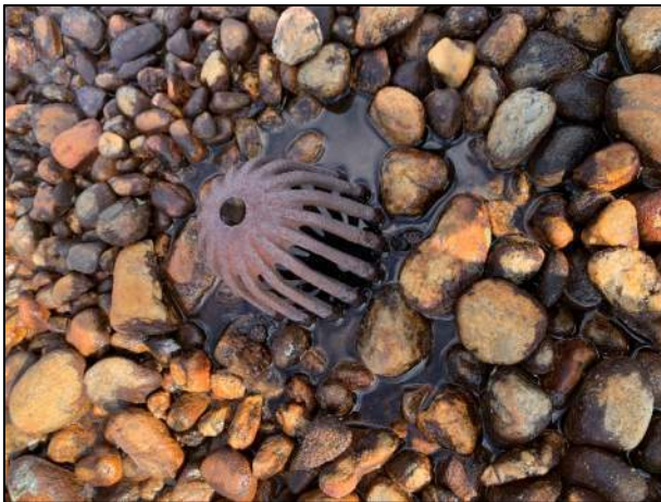
Figure 12: Clogged Roof Drain
