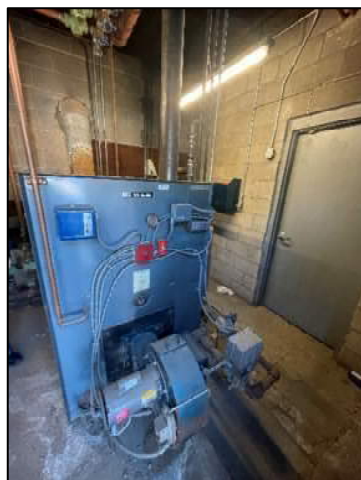
Figure 11: Gas-Fired Boiler in Shop Area
