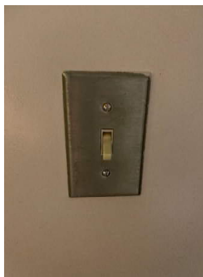
Figure 6: Toggle Switch
