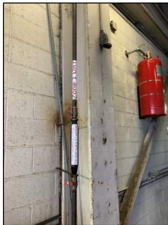
Figure 46: Dry-Chemical Suppression System
