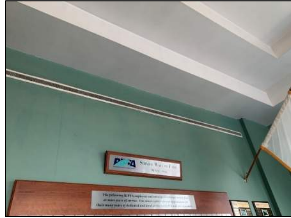
Figure 32: HVAC Diffuser in Lobby
