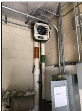
Figure 13: Electric Unit Heater in Water Room
