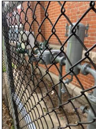
Figure 13: Gas Service Meter and Regulator
