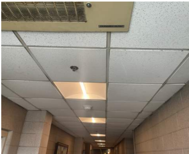
Figure 3: LED 2'X2' troffer fixtures
