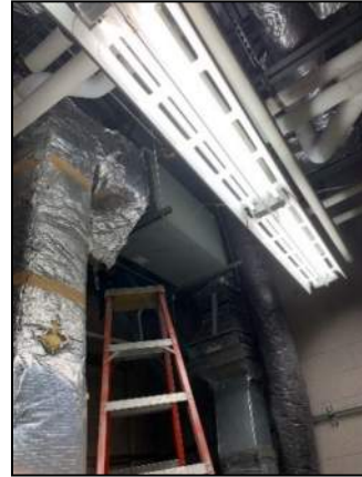
Figure 38: AC Fan Coil Unit
