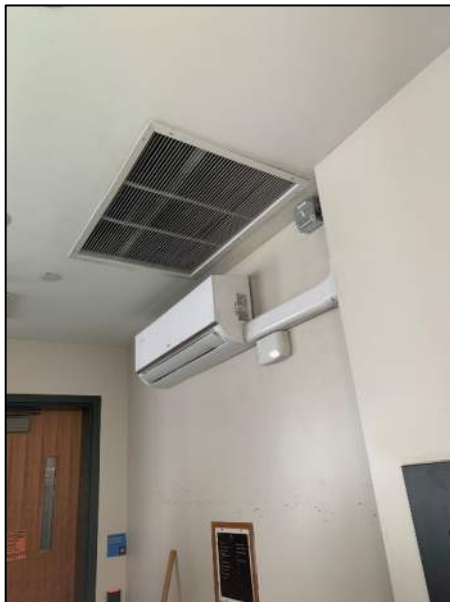
Figure 13: Wall-Mounted Indoor Unit in Dispatch Room
