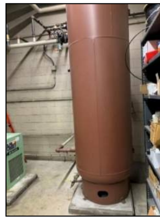
Figure 16: Compressed Air Tank
