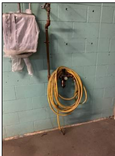
Figure 21: Compressed Air Drop
