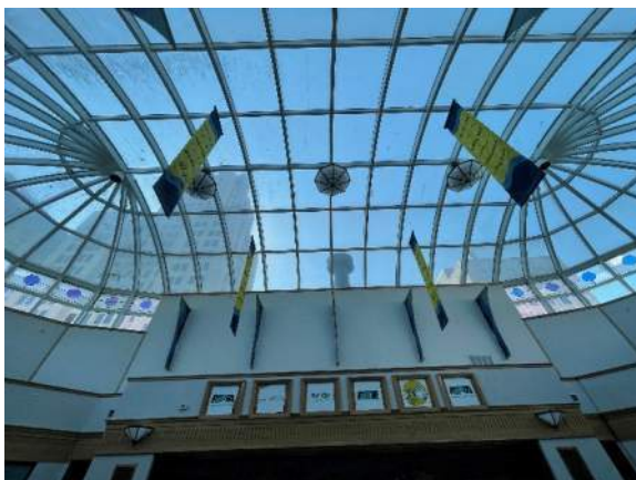
Figure 1: Decorative fluorescent pendants/wall mounted fixtures
