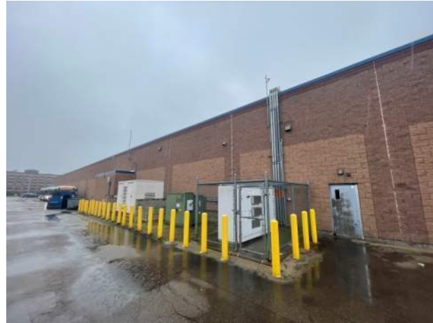
Figure 4: Transformer and Generator
