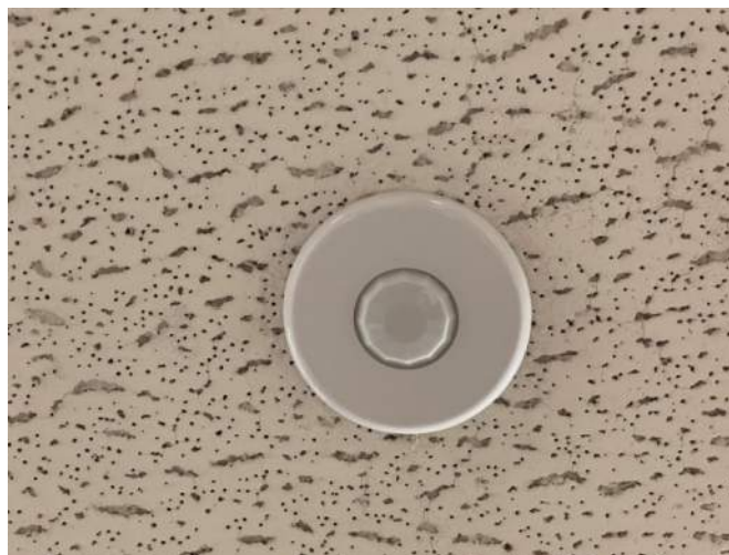
Figure 4: Ceiling mounted occupancy sensor
