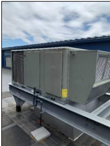
Figure 42: Roof Top Unit on Flat Roof
