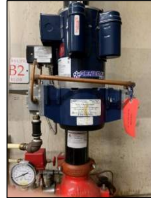
Figure 45: Riser-Mounted Air Compressor
