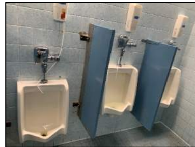
Figure 7: Touchless Operated Urinals
