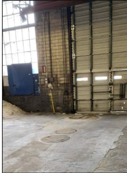
Figure 15: Filled Sand-Oil Separator
