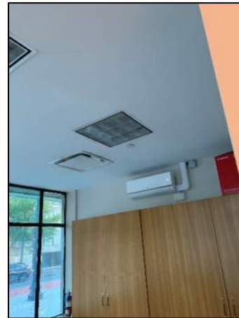
Figure 12: Wall-Mounted Indoor Unit
