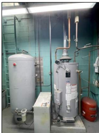
Figure 4: Gas-Fired Water Heater
