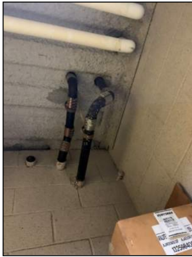
Figure 9: Sanitary Drainage Piping
