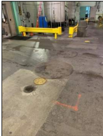
Figure 14: Oil Interceptors in Garage
