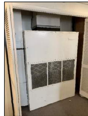
Figure 39: Indoor Evaporator
