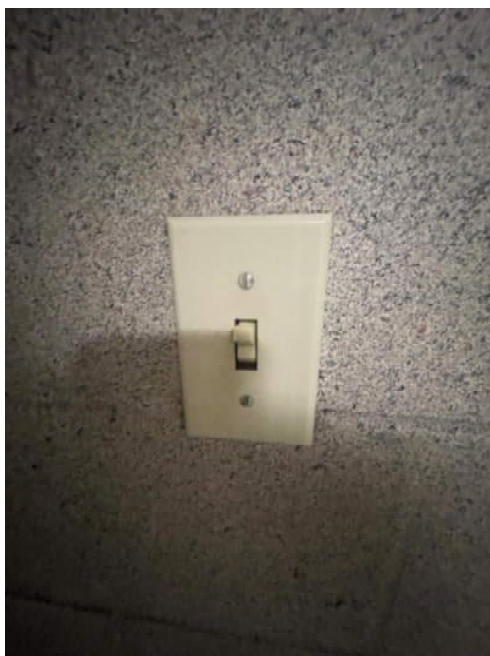
Figure 7: Toggle switches
