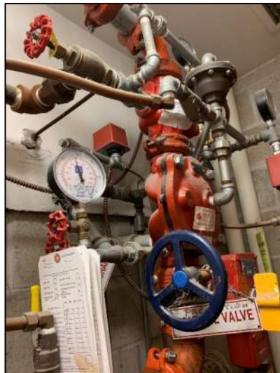
Figure 27: Pre-action System at Service
