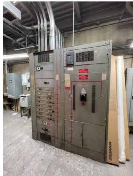
Figure 2: Switchboard (277/480V)
