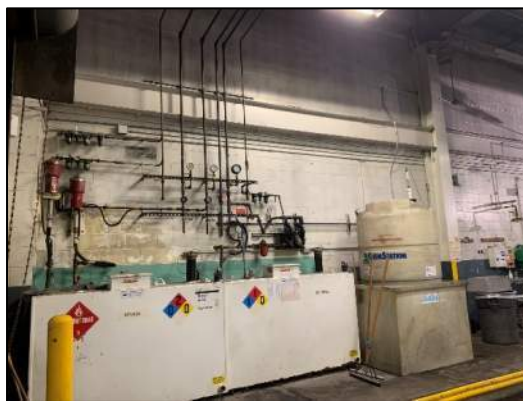
Figure 20: Lube System with Air-Operated Diaphragm Pumps
