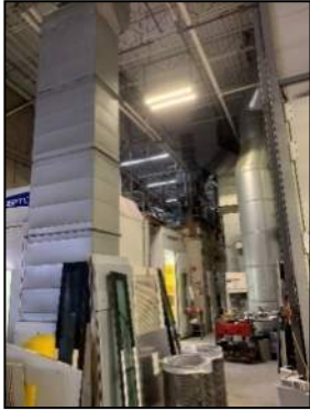
Figure 33: Paint Booth Exhaust System (Interior to Building, Exterior to Booth)
