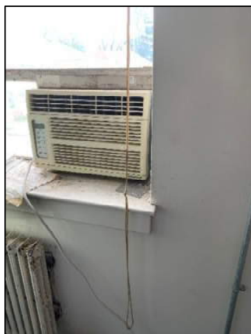
Figure 40: Window Unit in the Office Area
