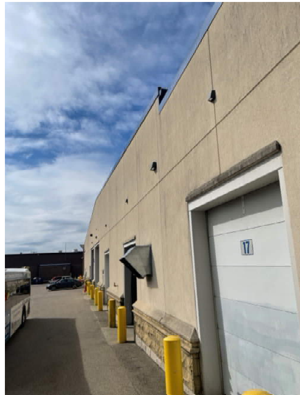
Figure 10: Emergency Wall packs
