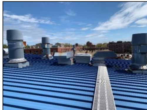
Figure 35: Paint Booth Exhaust Roof Terminations
