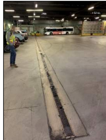
Figure 15: Trench Drain in Garage
