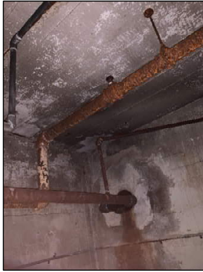
Figure 48: Rusty Fire Sprinkler Line, Basement
