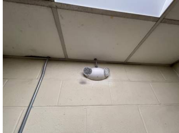
Figure 6: Emergency Battery Unit
