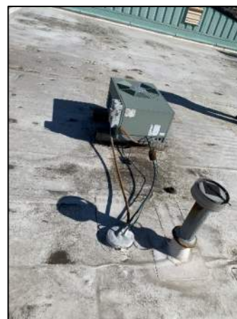
Figure 20: Roof-Mounted Condenser
