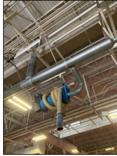
Figure 27: Localized Exhaust System Hose Reel
