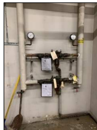
Figure 2: Non-Potable Water Backflow Preventers
