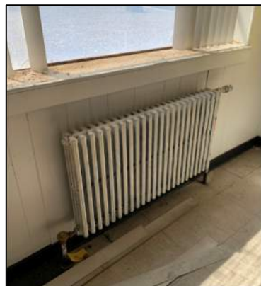
Figure 20: Steam Radiator in Breakroom
