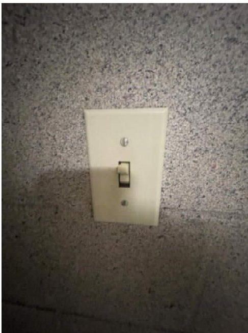
Figure 7: Toggle switches
