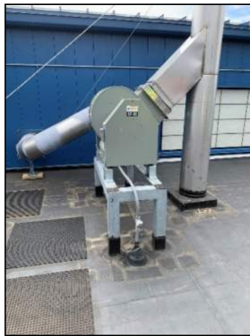
Figure 28: Exhaust Fan on the Roof
