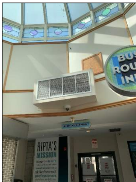
Figure 16: Diffuser in Concourse/Waiting Room
