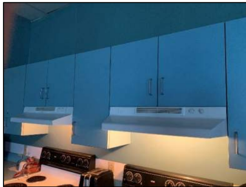
Figure 33: Recirculation-Type Hoods Over Stoves
