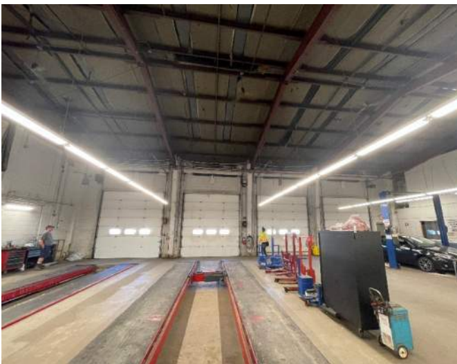
Figure 1: Fluorescent High-bay fixtures
