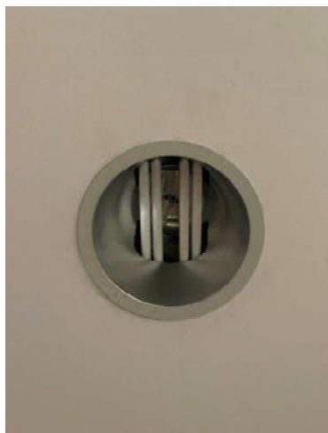
Figure 3: Fluorescent downlight fixtures
