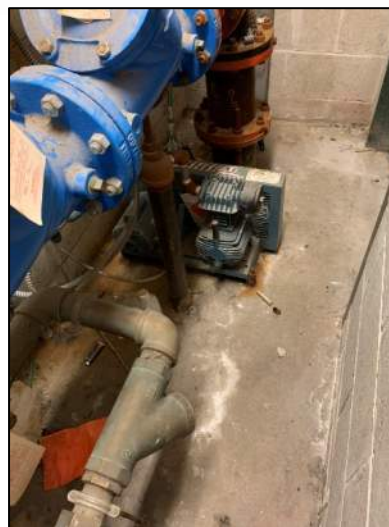
Figure 26: Air Compressor for Pre-Action System
