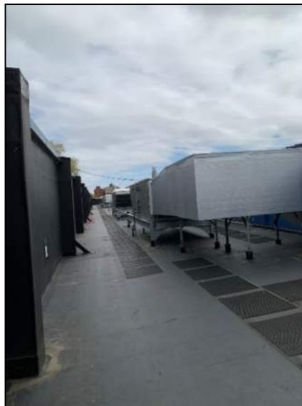
Figure 22: Makeup Air Unit Mounted on Roof
