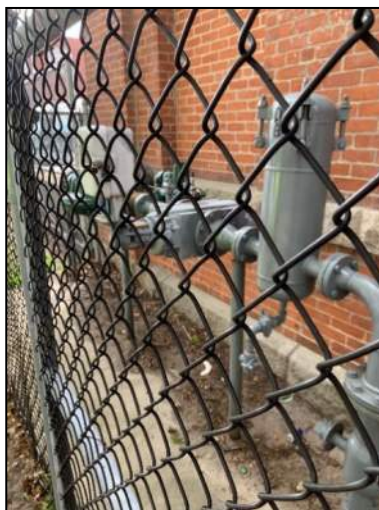
Figure 13: Gas Service Meter and Regulator
