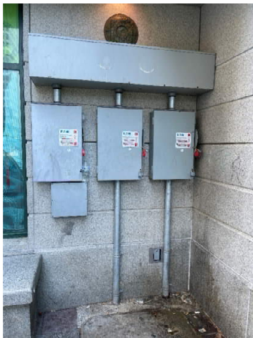
Figure 1: Main Service Disconnects
