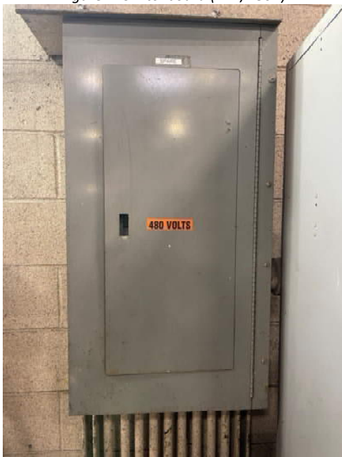
Figure 3: Abandoned/Damaged Panelboard
