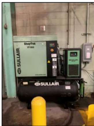
Figure 19: Compressed Air System
