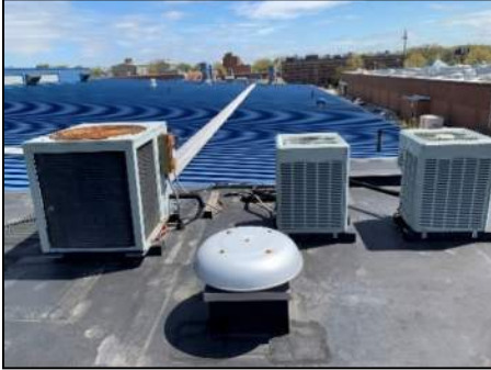
Figure 37: Air Conditioning Condensers on Flat Roof
