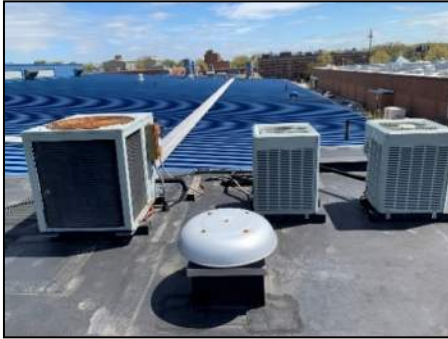
Figure 37: Air Conditioning Condensers on Flat Roof
