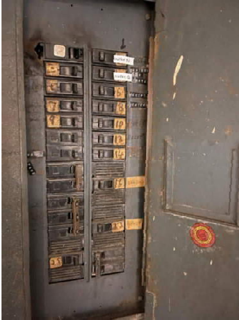
Figure 5: Deteriorating panelboard
