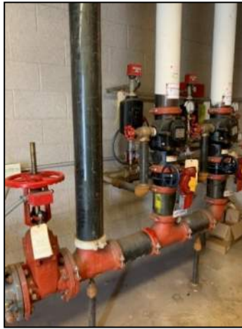
Figure 49: Fire Sprinkler Risers
