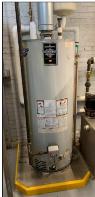
Figure 2: Gas-Fired Water Heater in Boiler Room
