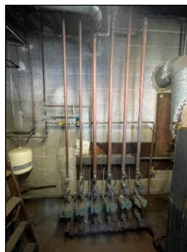
Figure 12: Hydronic Pump Manifold
