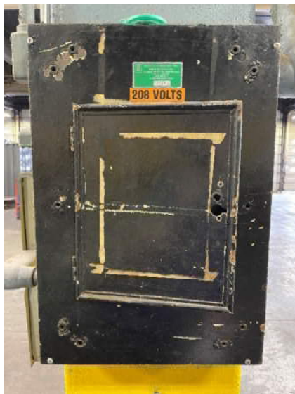
Figure 3: Deteriorating/Damaged Panelboard
