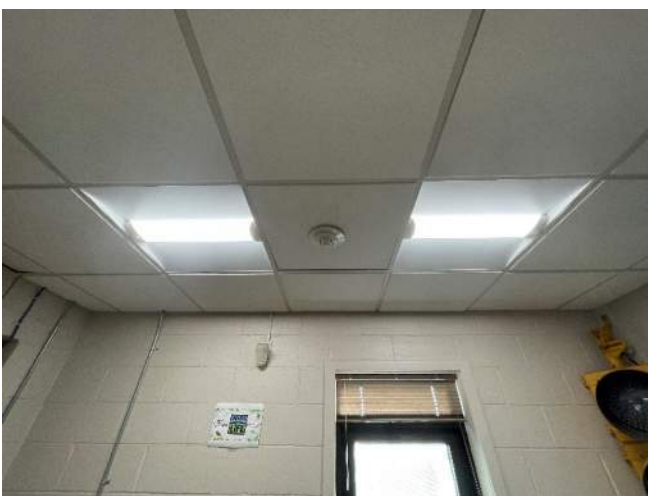
Figure 3: LED 2'X2' troffer fixtures
