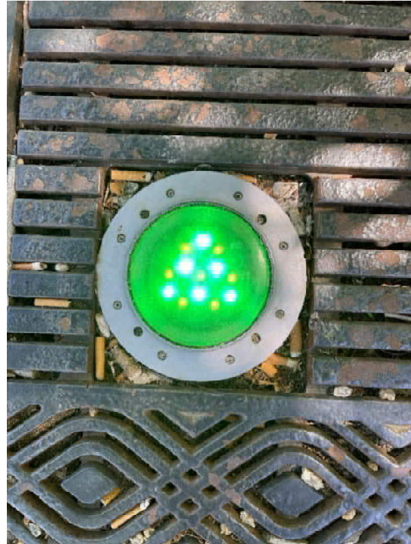
Figure 9: In ground LED RGB fixtures
