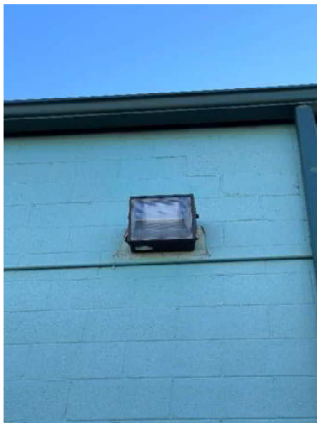
Figure 9: Exterior Wall pack
