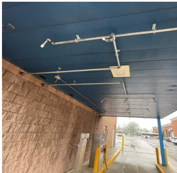
Figure 10: LED highbay under fuel canopy
