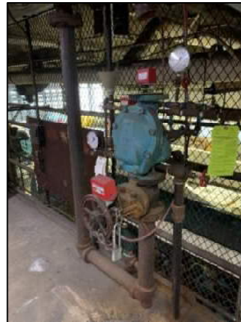
Figure 47: Abandoned Fire Sprinkler Riser
