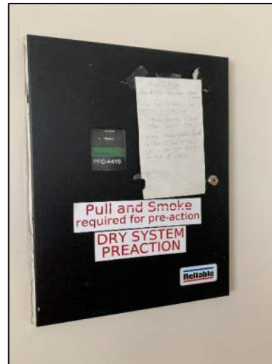
Figure 28: Pre-action System Controls
