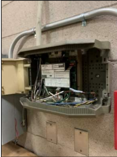
Figure 44: Abandoned BMS Control Panel
