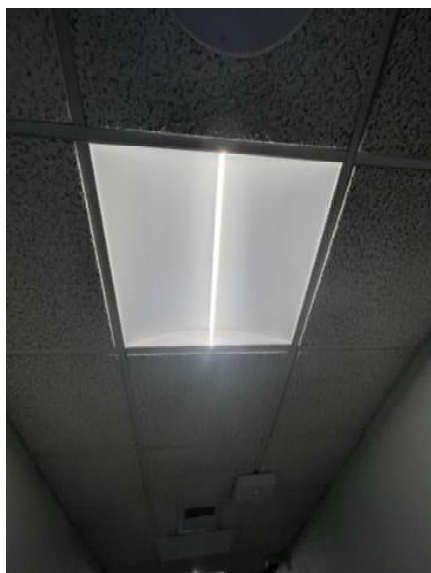
Figure 3: LED 2'X2' troffer fixtures
