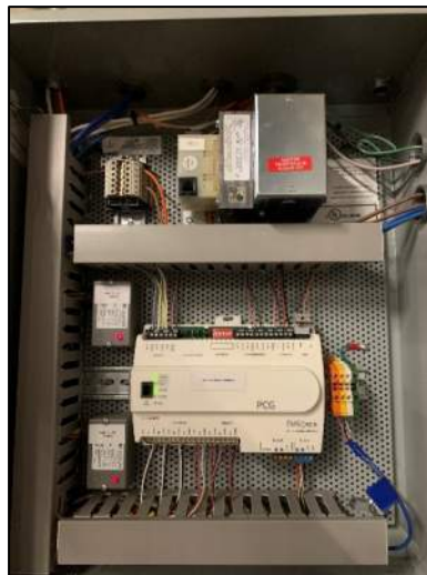
Figure 30: Johnson Controls BMS System Panel
