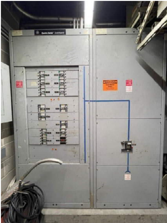
Figure 1: Switchboard (277/480V)
