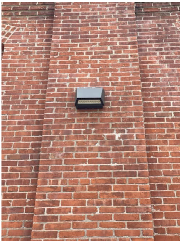
Figure 9: Exterior Wall pack
