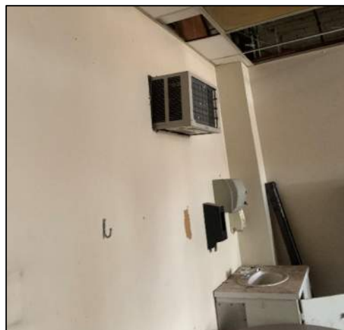
Figure 41: Window Unit in the Garage Area
