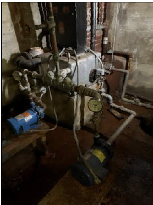
Figure 26: Condensate Receiver in the Basement
