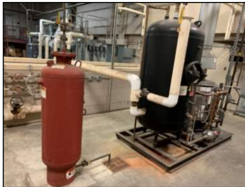
Figure 2: Domestic Water Boiler and Storage Tank
