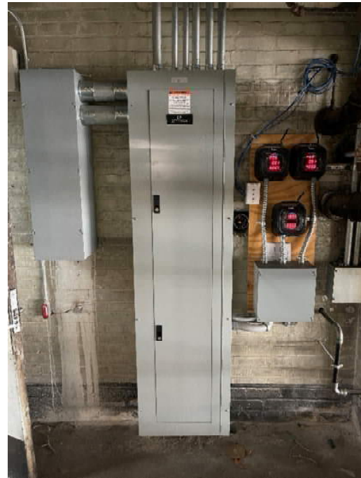
Figure 2: Main Distribution Panel 'DP' (277/480V)
