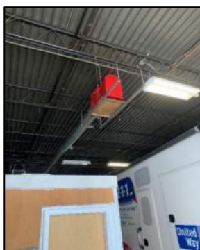
Figure 22: Exhaust Fan
