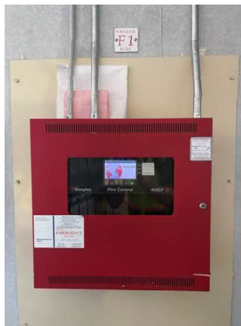
Figure 2: Fire Alarm Control Panel
