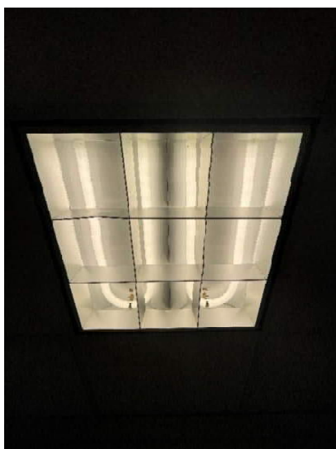
Figure 7: Fluorescent Fixture
