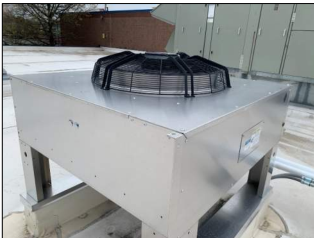
Figure 34: Condenser for Liebert System
