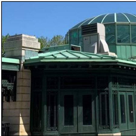
Figure 9: Rooftop Unit and Condenser for Split System
