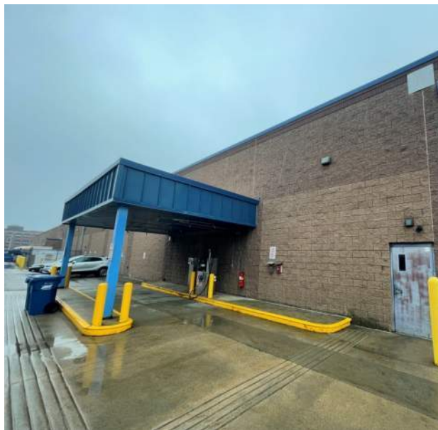
Figure 9: Exterior Wall packs and remote heads
