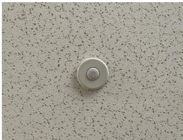
Figure 4: Ceiling mounted occupancy sensor
