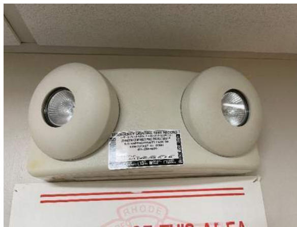
Figure 6: Emergency Battery Unit
