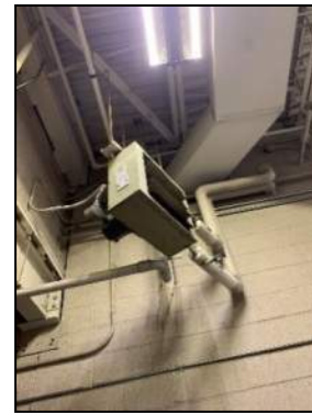
Figure 19: Hot-Water Unit Heater
