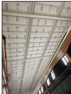
Figure 34: Paint Booth Exhaust (Interior to Booth)
