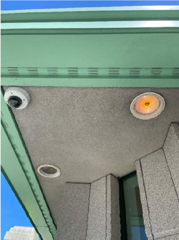
Figure 8: Exterior downlights
