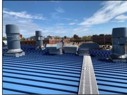
Figure 35: Paint Booth Exhaust Roof Terminations
