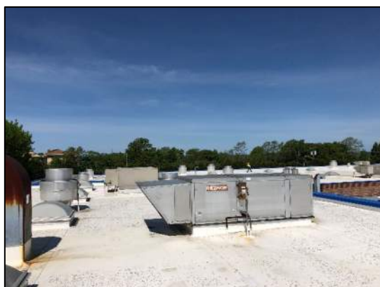
Figure 16: Makeup Air Unit
