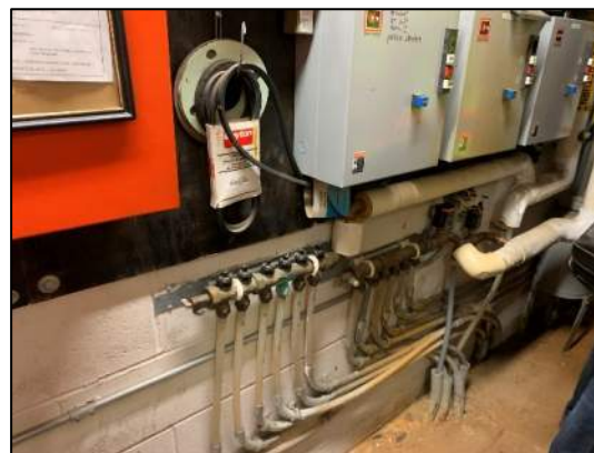
Figure 19: Radiant Floor Manifolds
