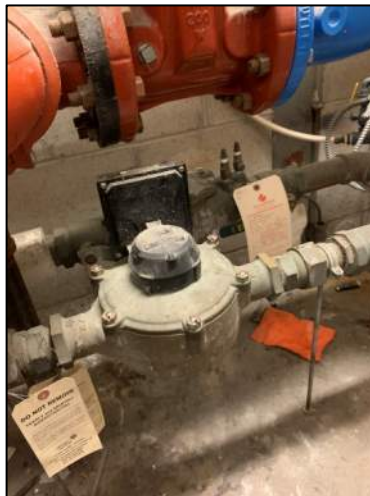
Figure 1: Domestic Water Meter and Backflow Preventer
