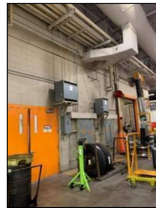
Figure 25: MAU Ducting from Garage to Surrounding Rooms
