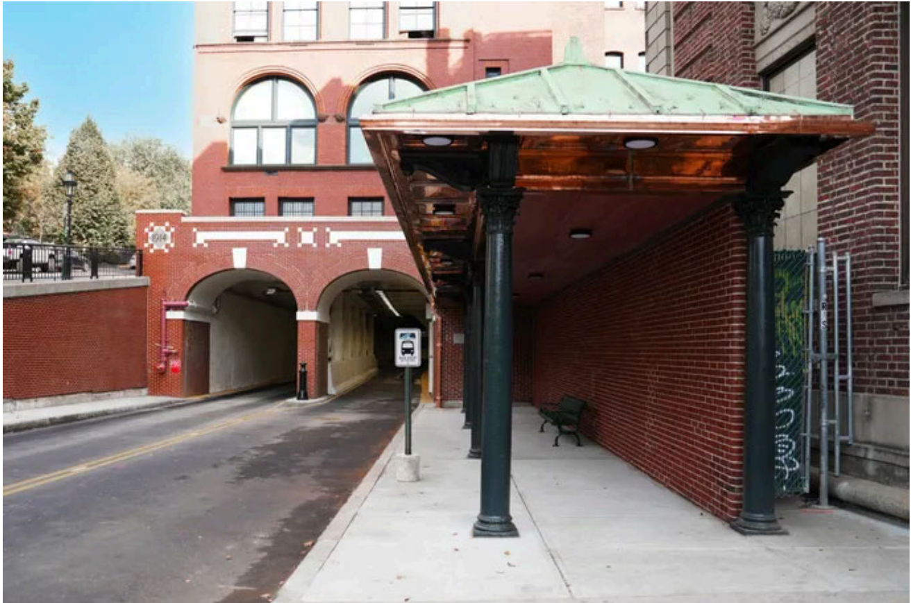
East Side Tunnel
